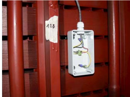
Fig. 3.: Sensor in a 128 MVA generator.
