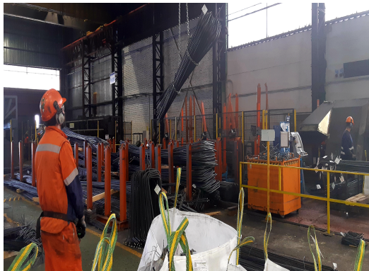
(a) Crane operator at work.
