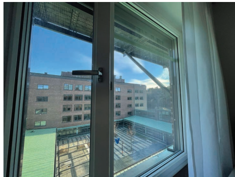
Figure 11.76 Photo of one of the A-building's triple pane windows and screens.
