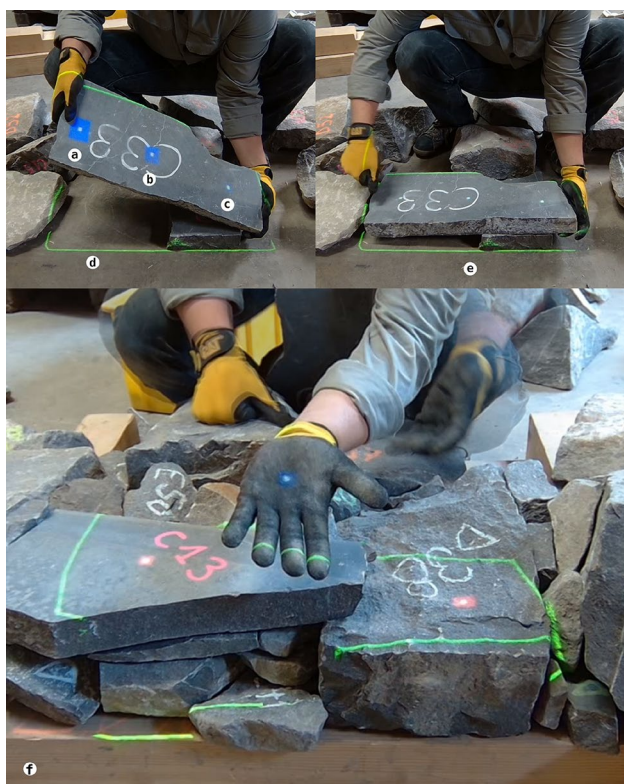
Fig. 13 Example of a stone placed with the proposed AR guiding framework: height probe (a) consistently, (b) moderately, and (c) close to the computed target, (d) UI widget to approximate the initial stone position, (e) interface state indicating a satisfactory pose. (f) To prepare a placement, the operator can also sense the targeted height indicated by each probe by inspecting the region with their hand. This haptic procedure allows the user to foresee the final height before start manipulating heavy building units
