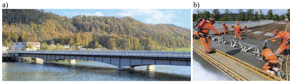
Figure 9. a) View of the steel-concrete composite bridge after R-UHPFRC strengthening, b) casting of UHPFRC with immediate application of curing compound.
