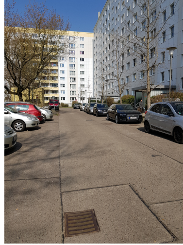
(b) Asphalt covered streets in the Slabs parcel
