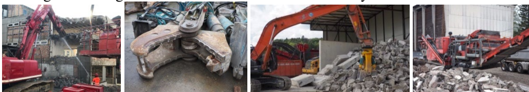
Figure 1. Tools and processes involved in the end of life of reinforced concrete.
