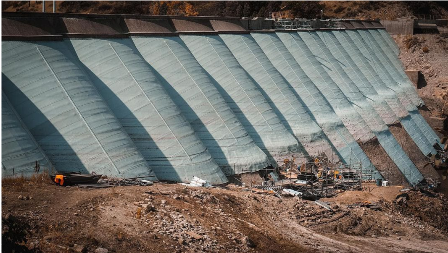
Figure 11: Dam rehabilitation in the USA. Image: courtesy of © Carpi Tech
