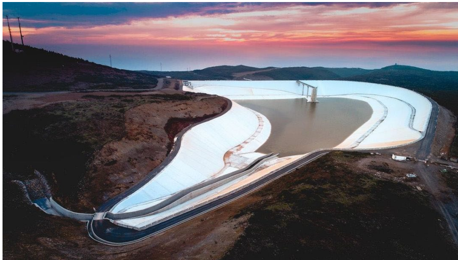
Figure 10: Geomembrane system in an upper reservoir in pumped-storage plant in Portugal. Image: courtesy of © Carpi Tech
