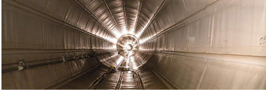
Figure 14: Geomembrane lining system in the US. Image: courtesy of © Carpi Tech
