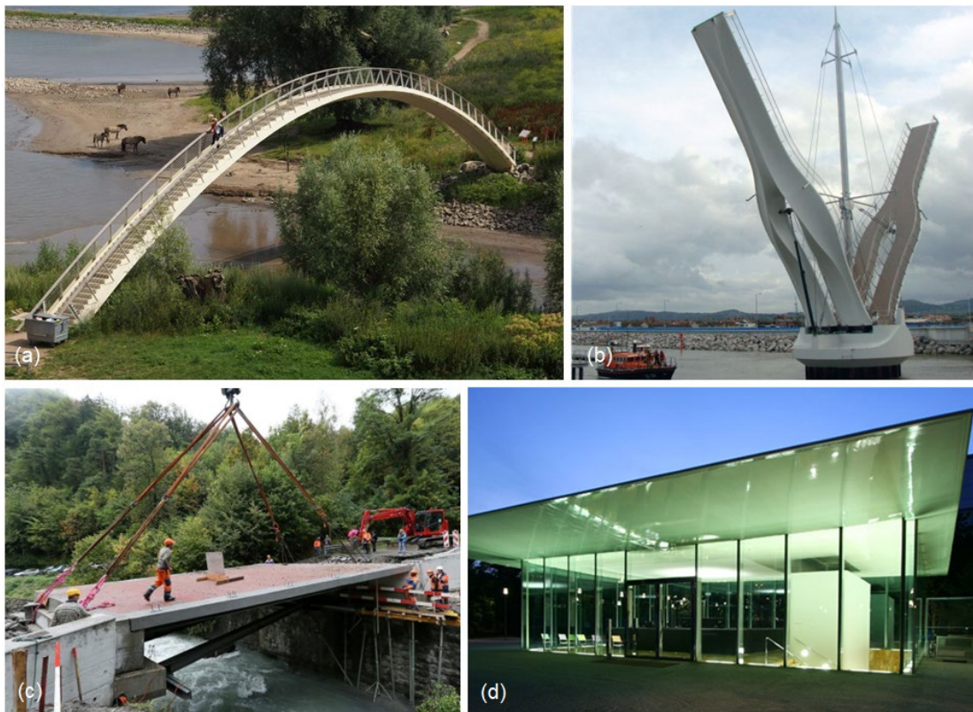
Fig. 1.1 Examples of composite constructions: (a) Ooypoort pedestrian bridge [12], (b) Pont y Ddraig [8], (c) Avançon bridge [9] and (d) Novartis Campus entrance building [11].
