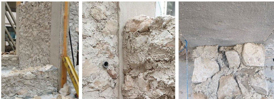
Fig. 6 Interface between the units in the stone masonry aggregate specimen
