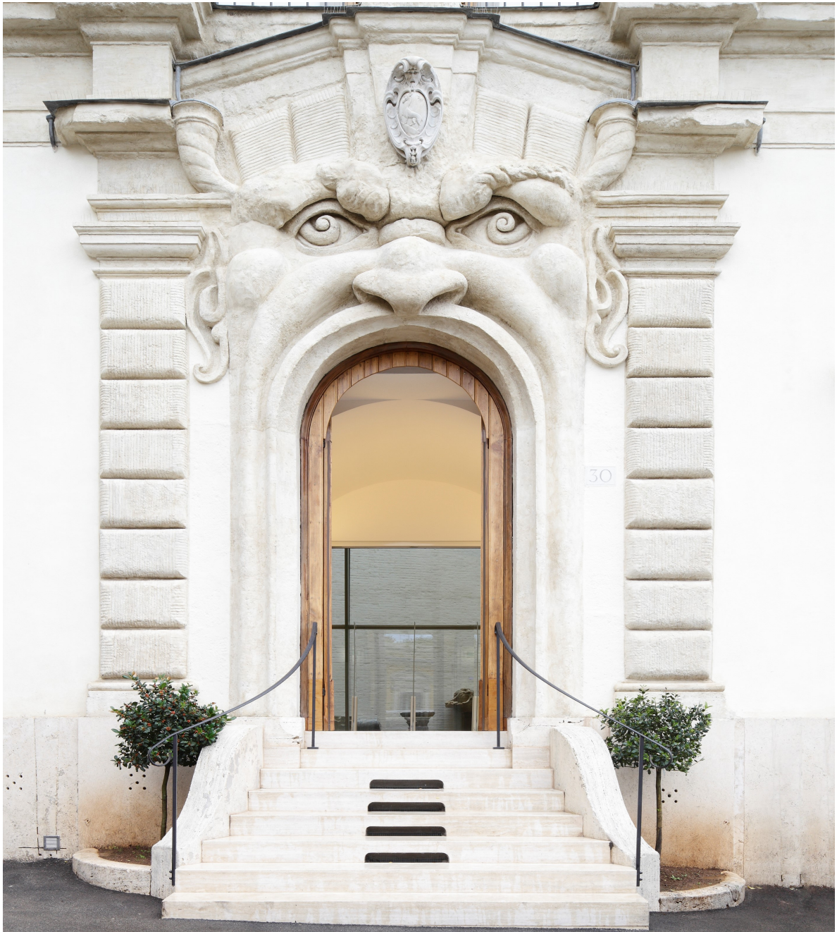
Figure 1.1: The mascherone entrance of Bibliotheca Hertziana on Via Gregoriana, which used to be the entrance to the garden of Palazzo Zuccari, now leads directly into the library. (Photo: Andreas Muhs)
