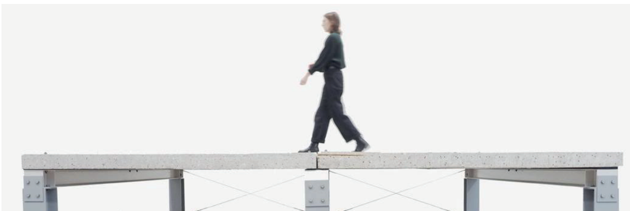
Figure 1. FLO:RE mock-up, made of reused reinforced-concrete and reused steel elements.
